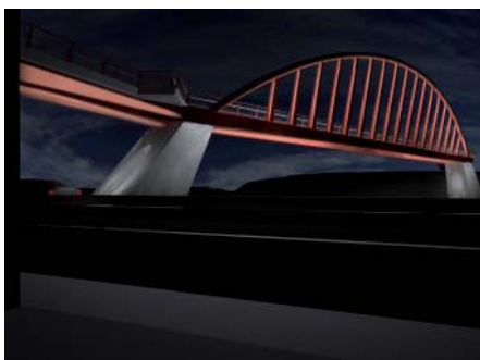
Puente peatonal East Hamilton, Ontario
