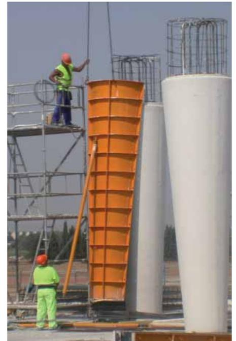
*The troncoconic pillar formwork removal*
