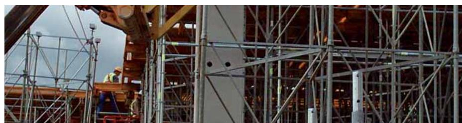
Close-up of the piece created by ULMA Construcción for moving the Shoring Towers.
