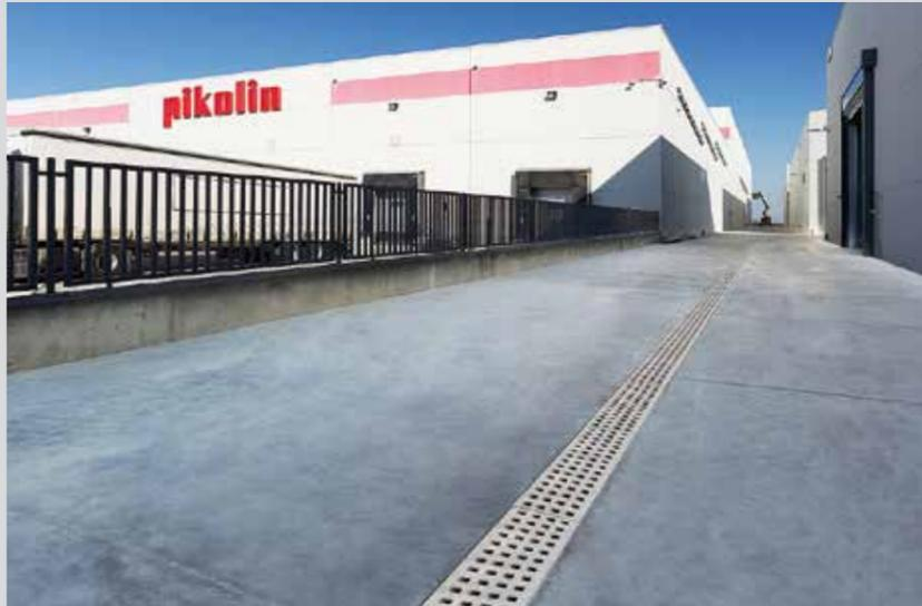
In total, **1910 linear metres of KOMPAQDRAIN® KVFD200.10R.E2530 Industry channels with a MAX FLOW® system were installed.** The channel has an innovative compact design and was manufactured with polymer concrete where the channel and the grating are one piece to ensure greater rigidity.
