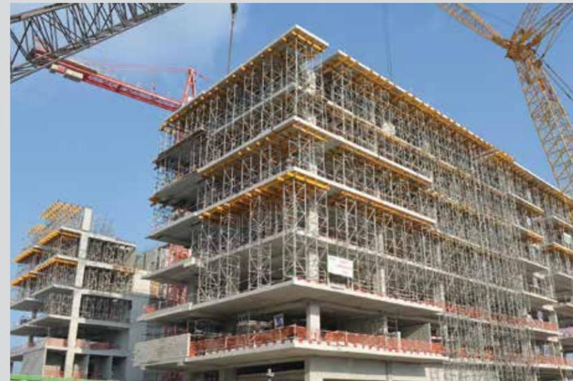
ULMA Construction has offered rapid, simple, and, most importantly, flexible solutions for this project composed of extremely diverse slab thicknesses and heights.
