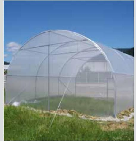
ULMA Agrícola product is 8 meters wide and more than 4 meters high with a 3.5 metre modulation between arches, which allows for a large open interior volume for crop culture.
