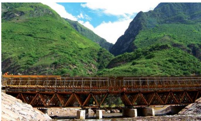
The MK BRIO scaffolding system, the NEVI formwork system and the 2000 Climbing Consoles were used in all the construction phases of the Tingo Bridge
