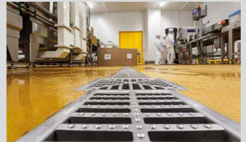
**MORE THAN 1,000 LINEAR METRES OF STAINLESS STEEL DRAINAGE HAVE BEEN INSTALLED IN THE LARGEST AND MOST MODERN MEAT PROCESSING PLANT IN EUROPE**
