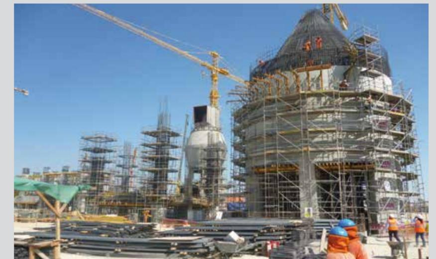
walls and easy to assemble, the brackets not only supported the COMAIN panels used as the formwork for the ring, but they also created a surface to which the working platforms could be attached, allowing the reinforcement and formwork to be installed.
