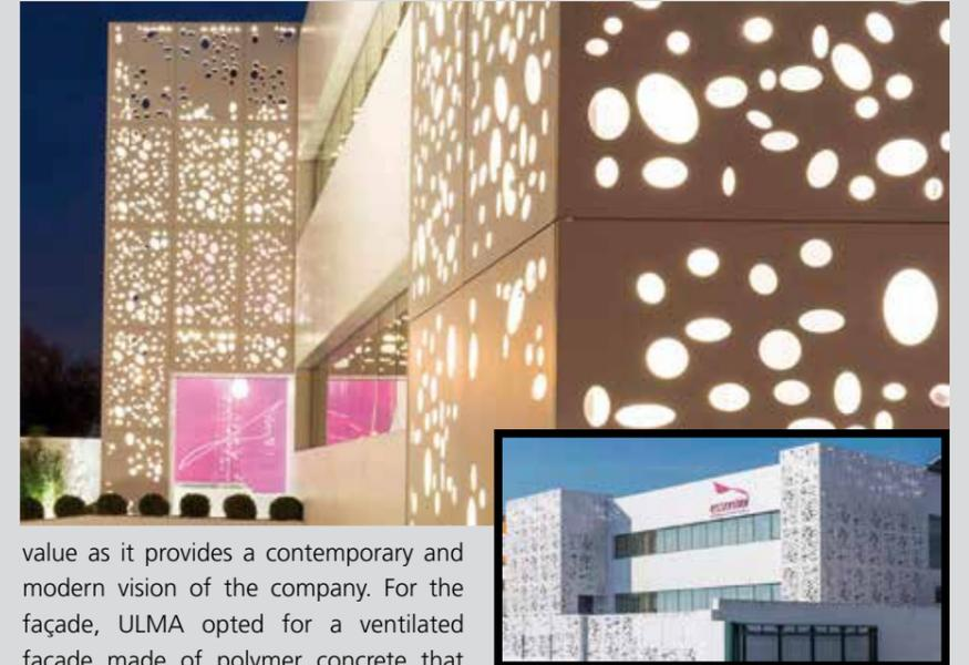
value as it provides a contemporary and modern vision of the company. For the façade, ULMA opted for a ventilated façade made of polymer concrete that creates volumes designed exclusively for this project. The purpose of this design was to convey the essence of the company based on the values of modernity and innovation.
