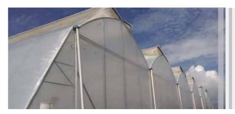
Among the good things of the G12 model by ULMA Agricola we can highlight the 12.8 meter wide span maximising the usable indoor space of the greenhouse The larger distance between pillars is compensated by the robustness achieved by the 90 mm oval profile in the arches, optimising the balance between volume and resistance.
