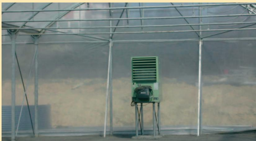
sary heating power has been obtained to achieve the desired thermal increase. In this way they can calculate the number of generators and the position in which to place them. The fuel for the installed generators is gasoil and has
