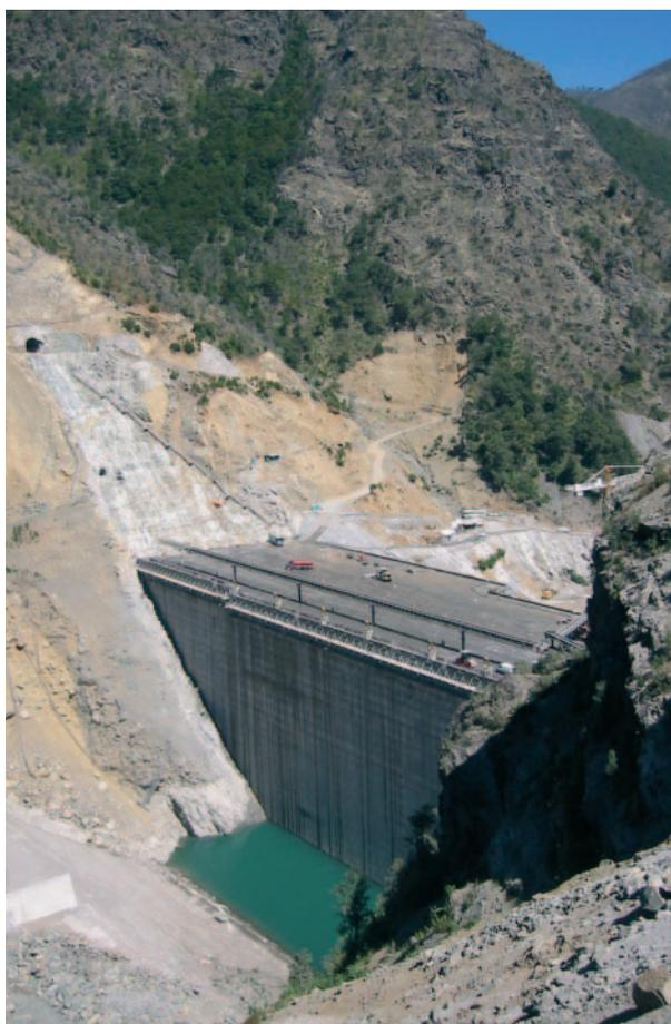
The hydroelectric complex is made up of three very defined parts: the dam, the lead in tunnel and the machine room. The reservoir contains 1,200 million cubic meters of water that feed the tunnel - seven kilometers long by nine meters in diameter. This takes the water to the machine room, where the two turbines and the generators that transform the hydraulic energy into electric energy are located.
