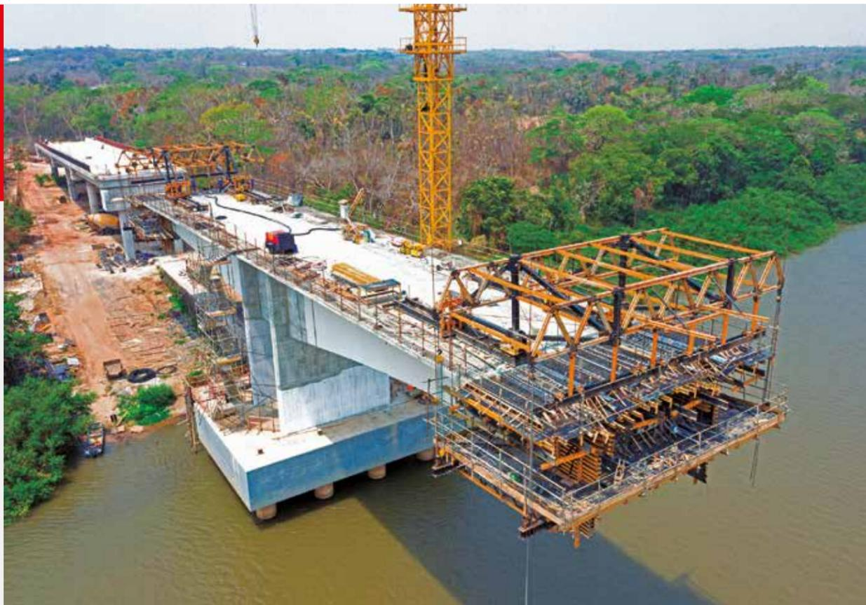
Construction is underway on a new bridge over the Cuiabá River in Brazil that uses the balanced cantilever method. The bridge will link the Parque do Lago in Várzea Grande with the Atalaia Park in the capital. The main challenge has been to avoid damage or disruption to the navigability of the river. The bridge is 390 metres long, with a span of 240 metres and 120 metres of navigable lane, through the central span, which takes account of the prerogatives of the Brazilian Navy.
