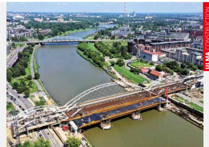
**Trusses**, 24 - 30 metres in length. This truss system is modular, requires minimal shoring, and is easy to assemble and handle. The narrowest span is made of 12 m long TAC steel profiles.
