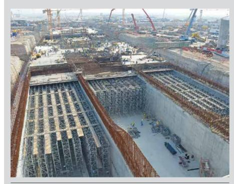
A CUT-AND-COVER TUNNEL 665M LONG AND 45M WIDE WITH THREE TUBES. THE CENTRAL TUBE IS FOR RAILWAY TRAFFIC WITH TWO LINES IN EACH DIRECTION.
