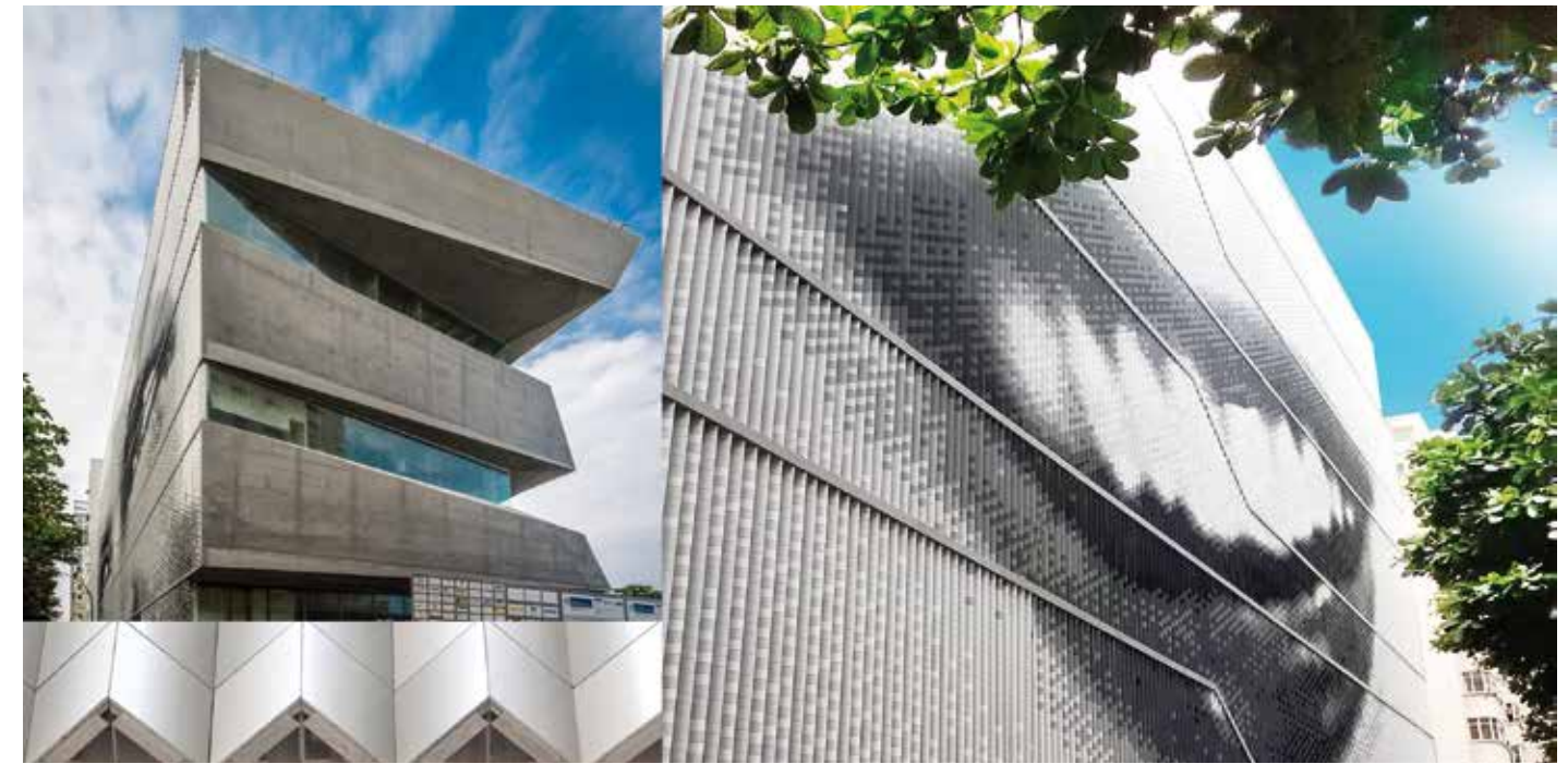
>> Photo showing the location of the building’s western facade, detailing the montage of the plates and one of the mural’s two views
