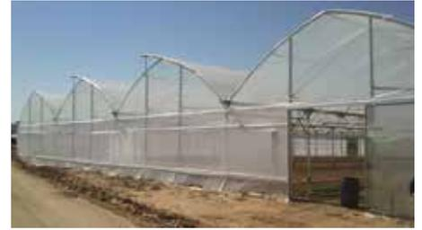
more technical and professional and ULMA Agrícola has participated in this process installing the first Multi-chapel Gothic type greenhouse to cover nearly 4,000 square meters equipped with super-zenith ventilation and rollup perimeter ventilations to facilitate the renovation of air inside the greenhouse.
