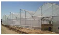
more technical and professional and ULMA Agrícola has participated in this process installing the first Multi-chapel Gothic type greenhouse to cover nearly 4,000 square meters equipped with super-zenith ventilation and rollup perimeter ventilations to facilitate the renovation of air inside the areenhouse.
